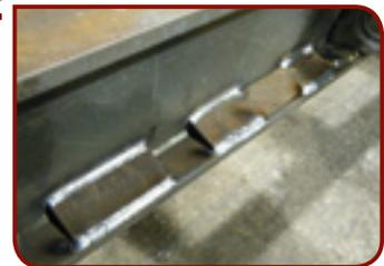
Reinforced Top Flange (Underside View)
