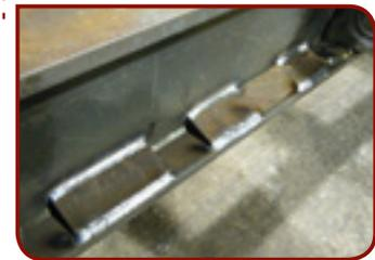
Reinforced Top Flange (Underside View)
